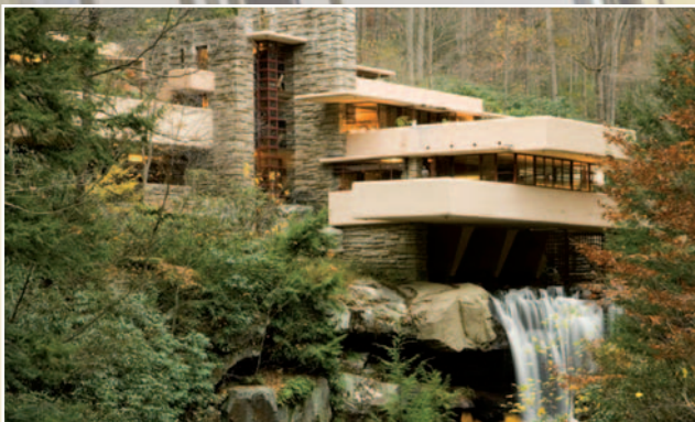
4) Falling water, F.L. Wright
